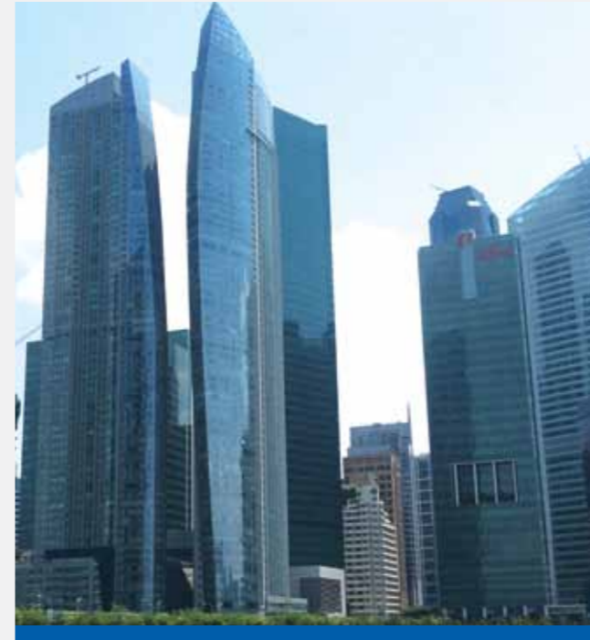
THE SAIL @ MARINA BAY FLOORING SYSTEM
