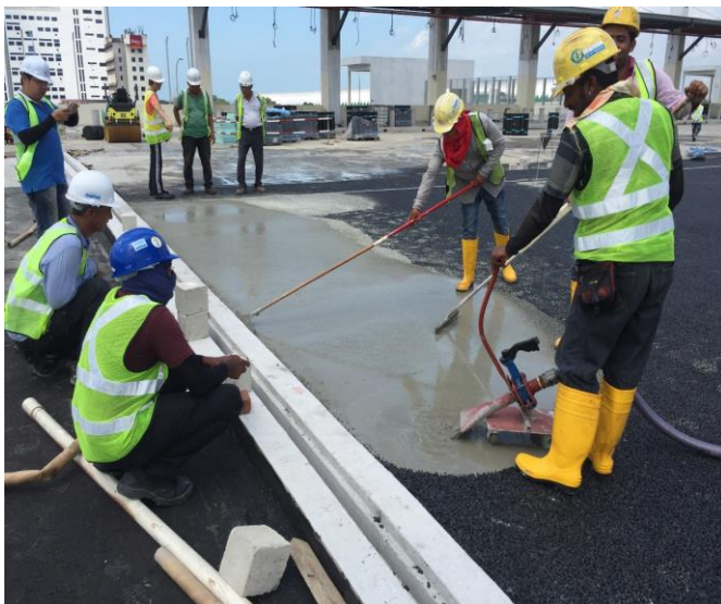
Semi-Rigid Pavement (SRP) Construction in Progress, Singapore, 2016
