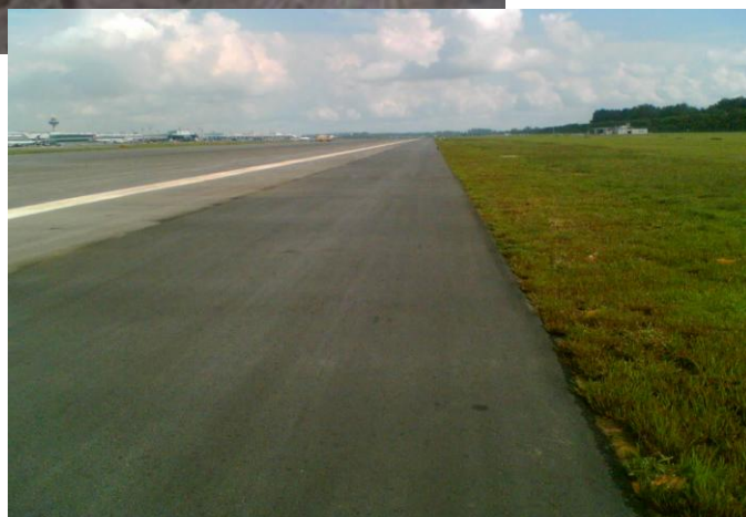
Singapore Changi International Airport Runways Widening, 2005
