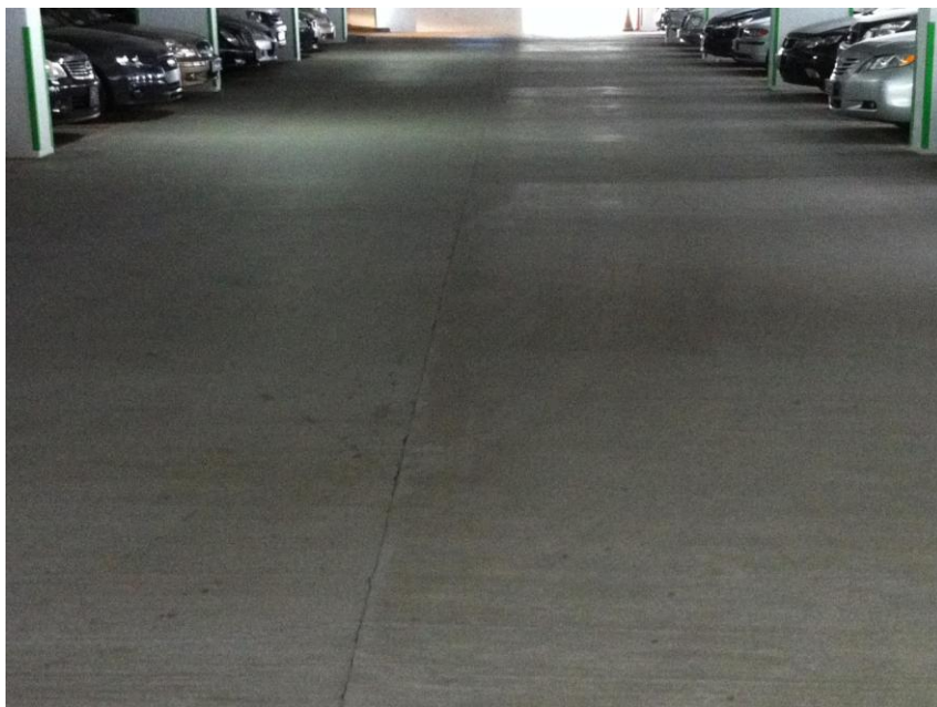
Multi-Storey Car Park at Chin Swee Road, Singapore, 2011
