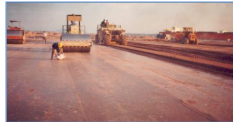
b) In-Situ Mixing and Compaction
