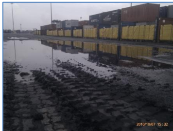
a) Before Upgrading
