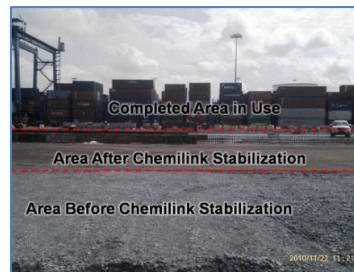
b) Before and after Stabilization
