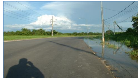
Photo. 10. A Stabilized Road at Low-Lying Area (2004)
