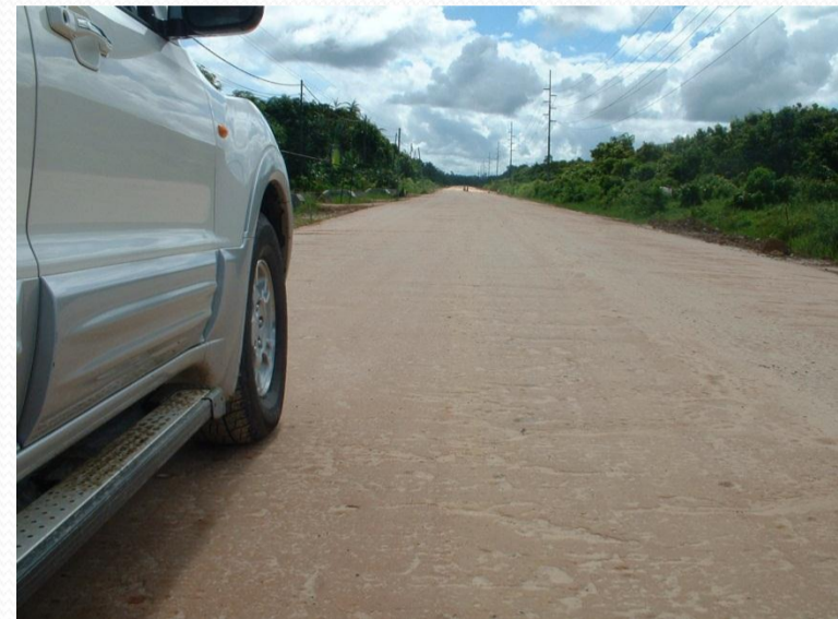
Mixture after Paving and Compaction
